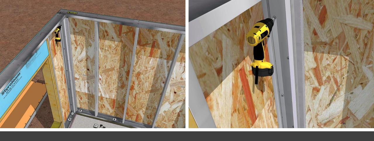
Set up your first corner to provide support to the first wall to be erected.
