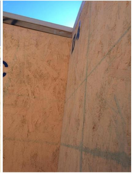
Attach first row of 2x6" Cap Plates by screwing from underneath top section of SuperPanel into Cap Plate.
