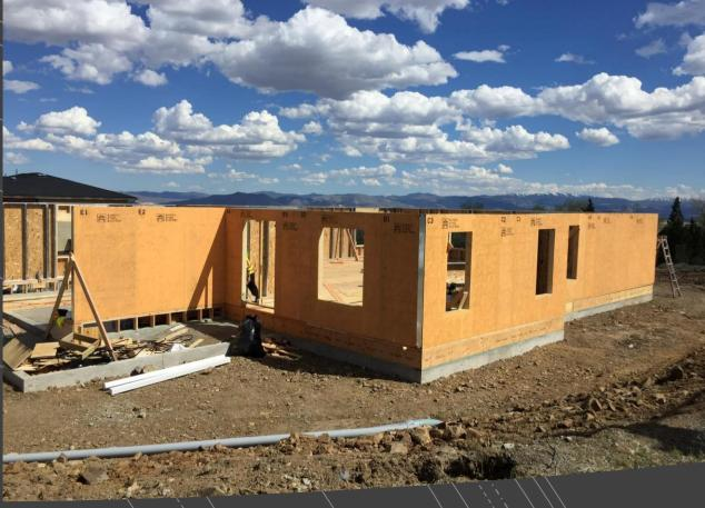
What we carefully pre-build at our factory, makes the onsite build a much-improved process that significantly benefits both the builder and end user. Whether a slab on grade or wood foundation system the SuperPanel is bolted firmly through the sill plate in the same manner used in old fashioned wood framing
